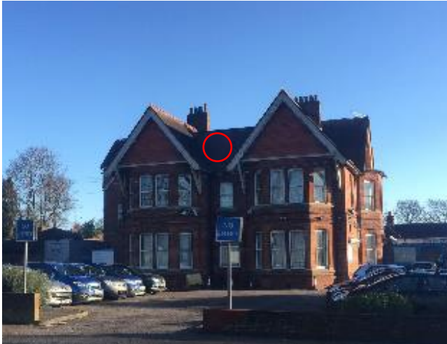
Roost access A (one common pipistrelle)
