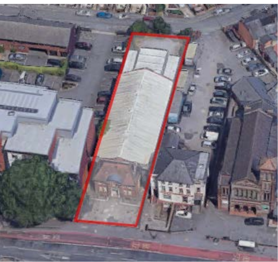
FIG 06 - AERIAL CLOSE-UP - SOUTHERN VIEW The site boundary extends from King's Road at the front (south facing) to Norwood Road to the rear (north facing). The existing swimming pool building fills the majority of the site width. The pool flank walls (to be demolished) informs the extent of the proposed building footprint. A low level retaining wall forms the boundary to the adjoining sites to the east and west.
