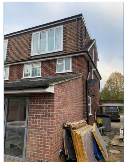
2. Rear and side of 12 Falmouth Road. Photo provided by the agent on 13/10/2020.
