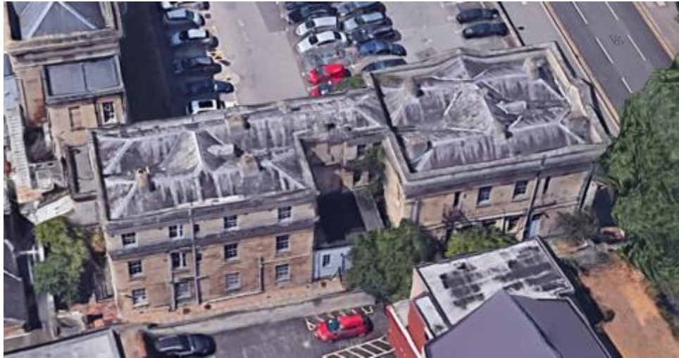
Google maps 2D aerial image from the eastern side showing the narrow link and infill, the complex hipped roof structure, and some surviving chimney stacks but much reduced in height and/or capped off
