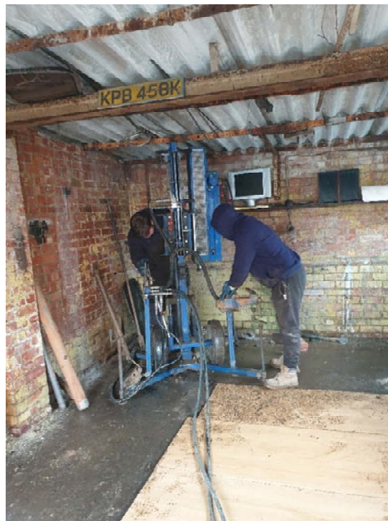
Photograph 6: Setting up the drilling rig at BH2
