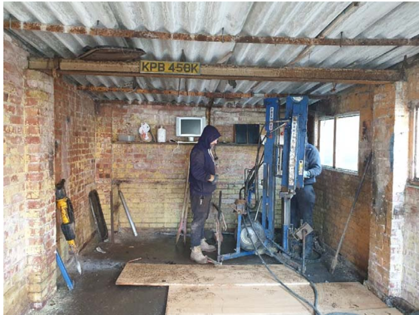
Photograph 1: A view showing the drilling rig set up at BH1 located to the rear of the garage
