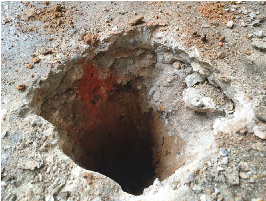
Photograph 7: A view showing the thickness of concrete, gravel sub base and sands beneath
