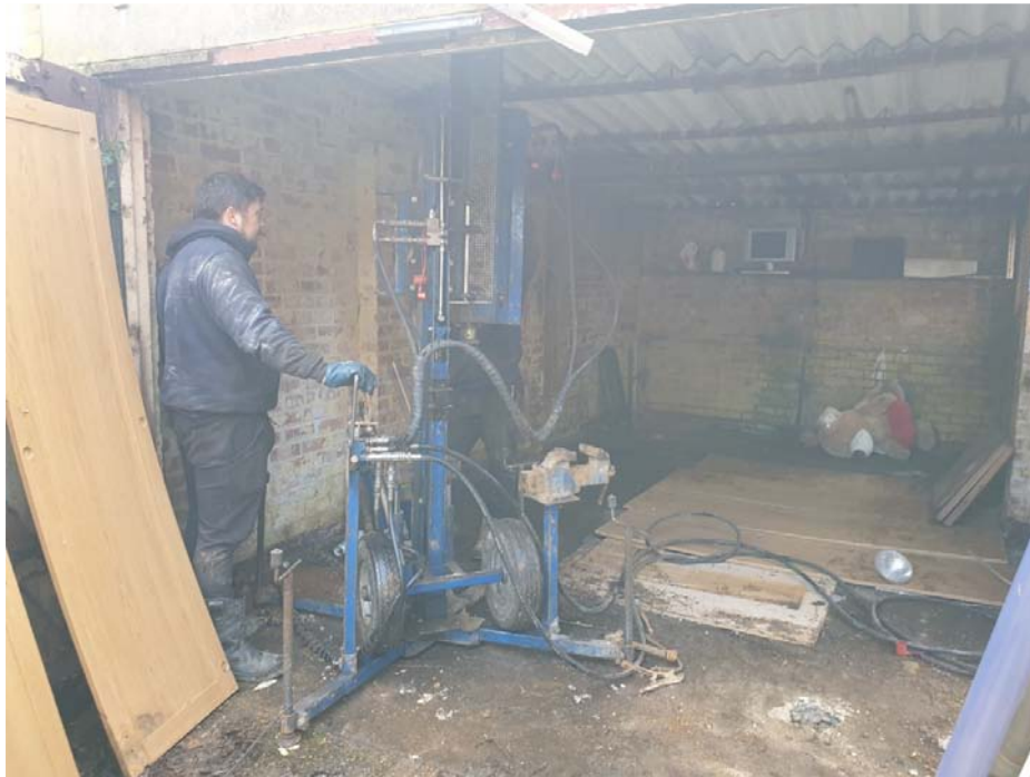
Photograph 10: Setting up at BH3.
