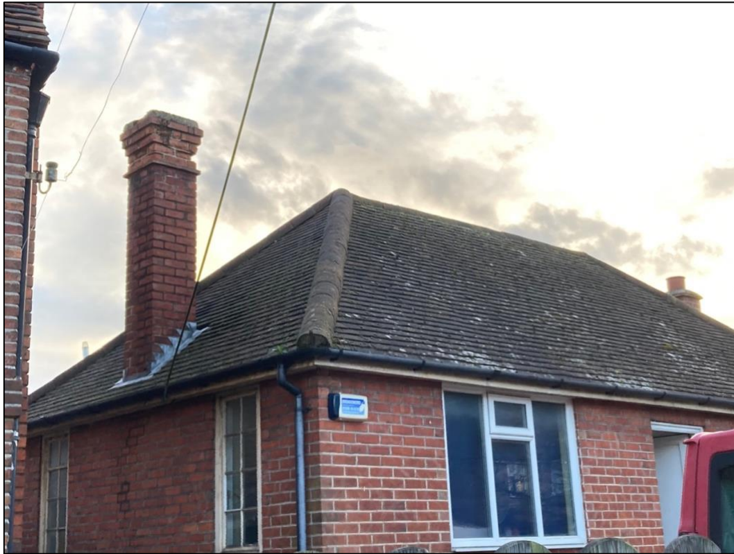
Photograph 7. The northern (front) and eastern (side) elevation of the bungalow at 389 Gosbrook Road showing the majority factory made clay tiles with negligible bat roosting potential.
