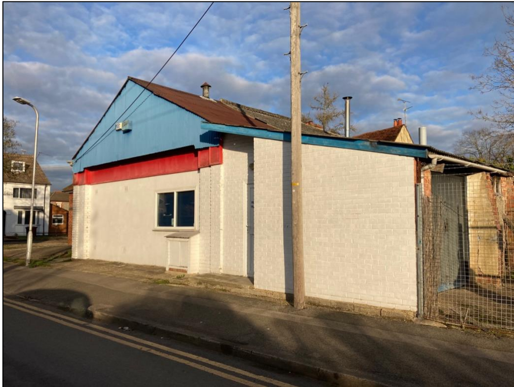
Photograph 3. The western (side) elevation of the workshop at 389 Gosbrook Road.
