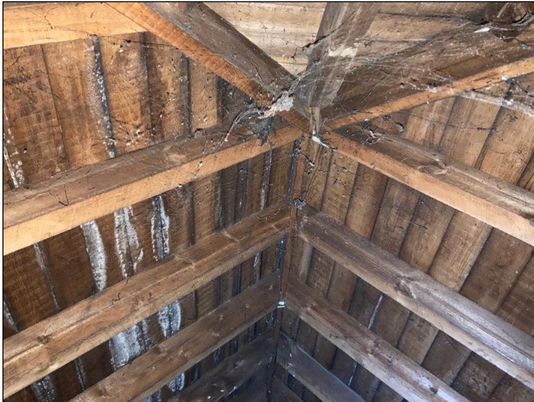
Photograph 9. The loft void within the bungalow at 389 Gosbrook Road showing the heavily cob-webbed timber beams, timber frame and roof lined with close-boarding.
