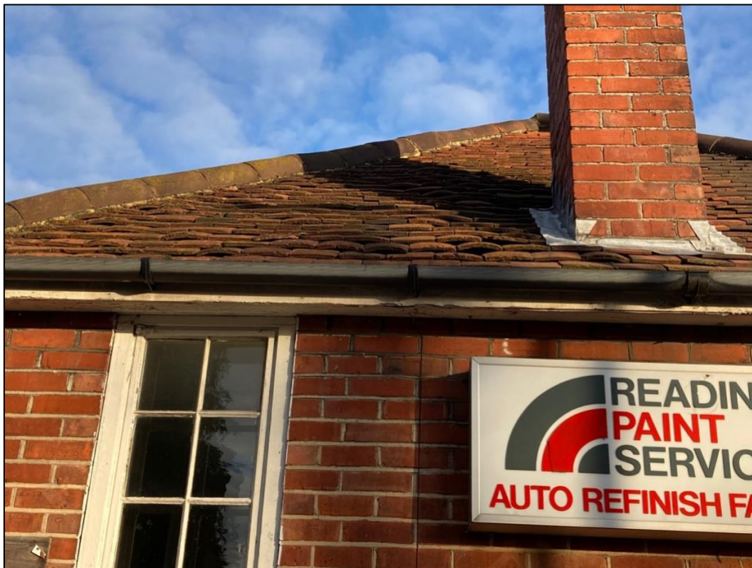
Photograph 6. The western (side) elevation of the bungalow at 389 Gosbrook Road showing potential bat access and roosting features between hand-made clay roof tiles.
