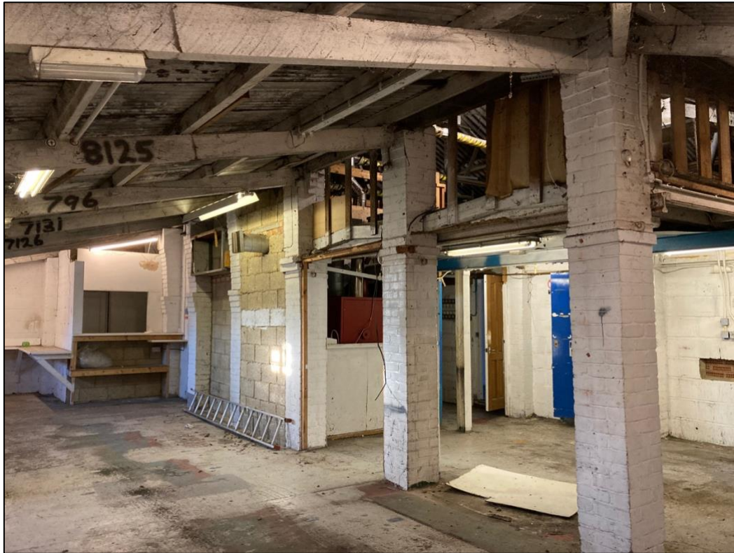
Photograph 13. The internal areas of the workshop at ground-level.
