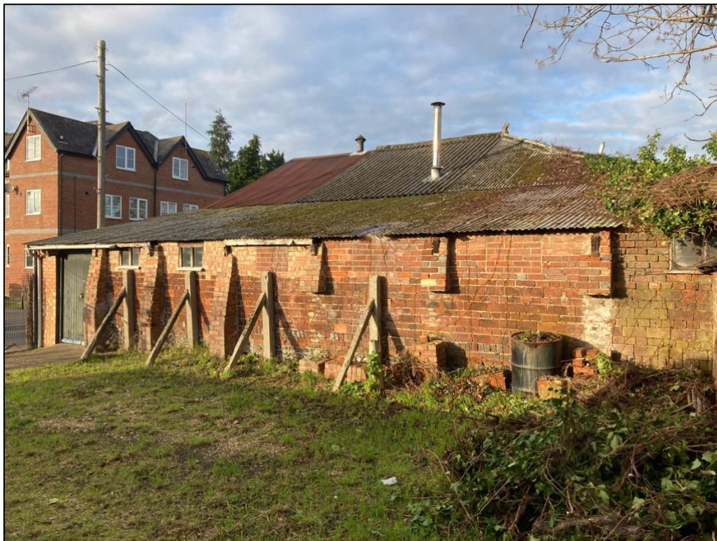
Photograph 4. The southern (rear) elevation of the workshop and part of the yard at 389 Gosbrook Road.
