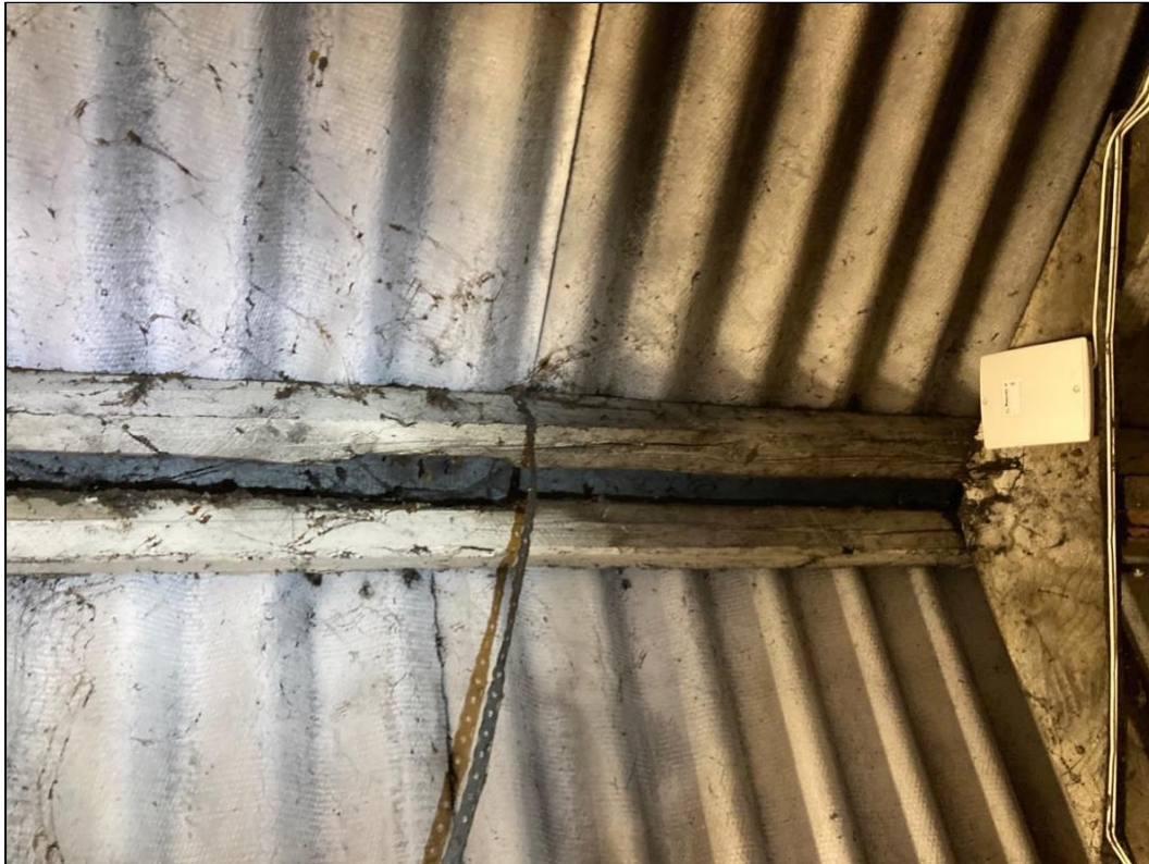
Photograph 11. Showing the underside of the apparent gap feature created at the ridge, highlighting that internally there is an absence of a crevice-feature suitable for use by roosting bats.
