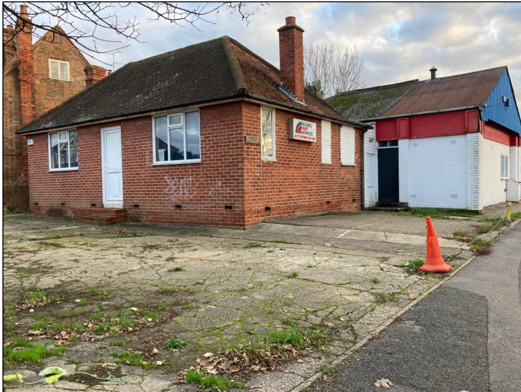
Photograph 1. The northern (front) and western (side) elevation of the bungalow and workshop at 389 Gosbrook Road.
