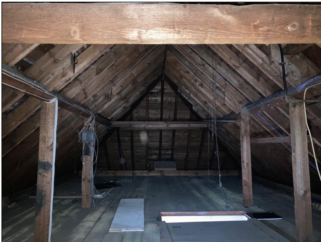
Photograph 8. The loft void within the bungalow at 389 Gosbrook Road showing the boarded floor, timber frame and roof lined with close-boarding.
