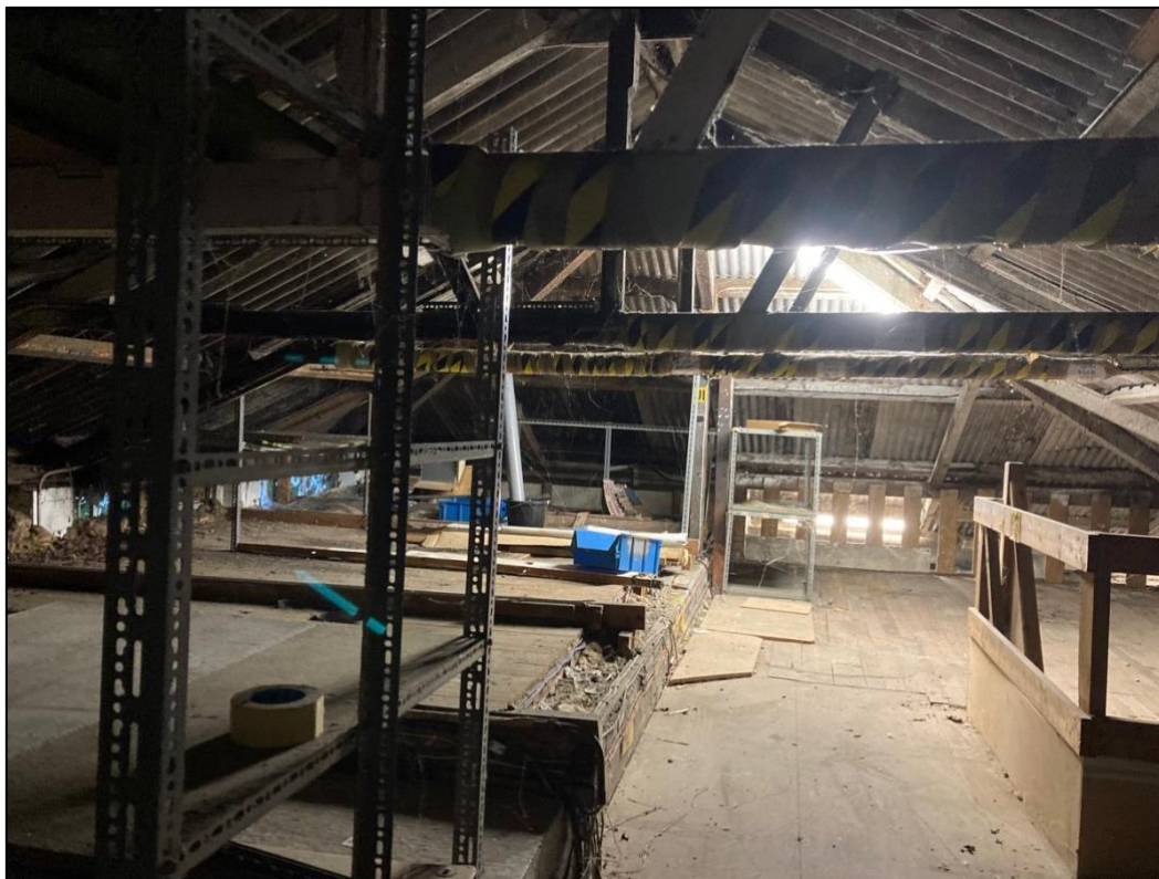
Photograph 13. The internal areas within the raised storage area of the workshop.
