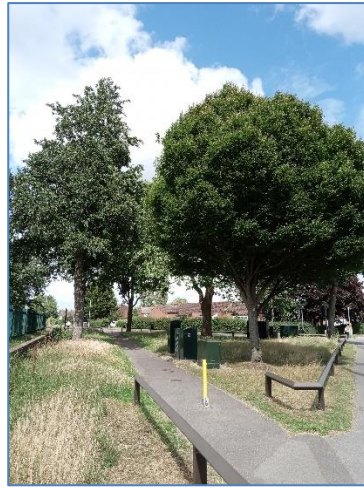
Fig 8. Existing cabinets next to proposed equipment location.
