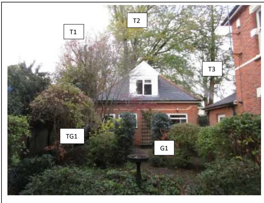
View of garage from rear
