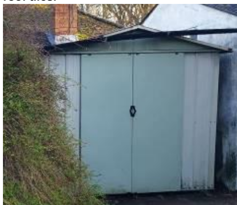
4. Simple corrugated shed (B3) to the rear of the garage.
