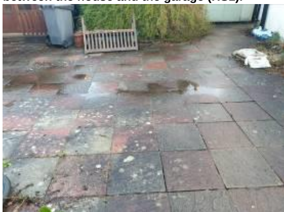
5. Large patio to the rear of the bungalow (HS2).
