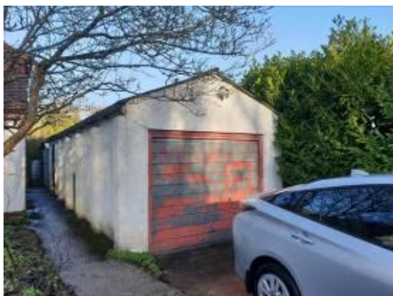
3. Detached garage (B2) with corrugated roof sheeting; concrete driveway and pathway between the house and the garage (HS1).
