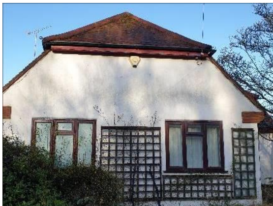
1. The front elevation of the bungalow, featuring a half-hipped eastern gable (B1).
