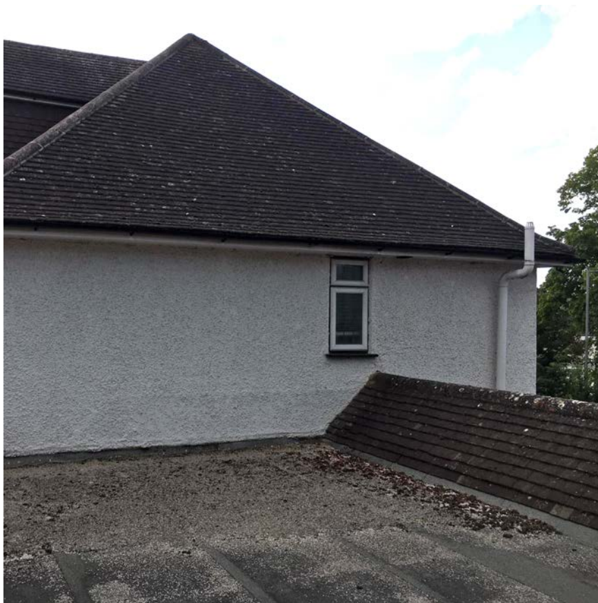
Figure 10 - Window currently overlooking 33 Cadugan Place
