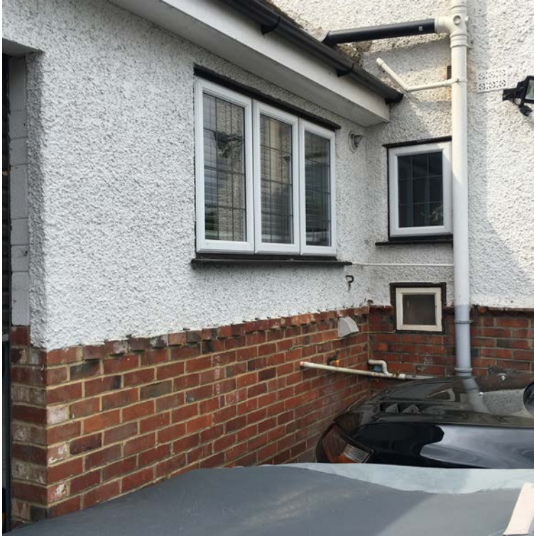
Figure 3 - The junction where the brickwork of the original house and new extension is visible at the side of the property.
