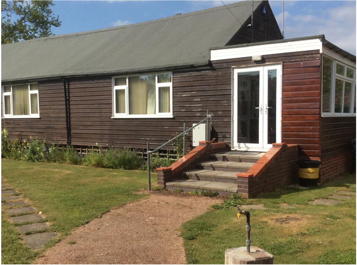
Existing Clubhouse - Elevated Above Flood Level
