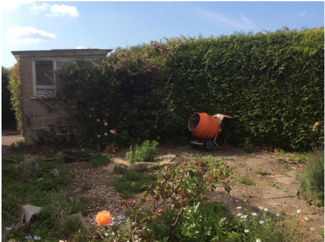
Site of New Temporary Building
