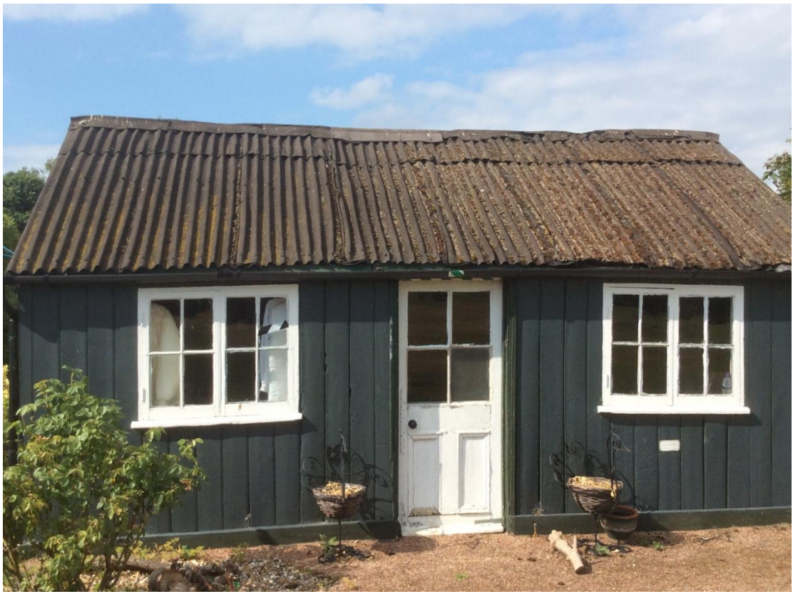
Existing Building to be Replaced
