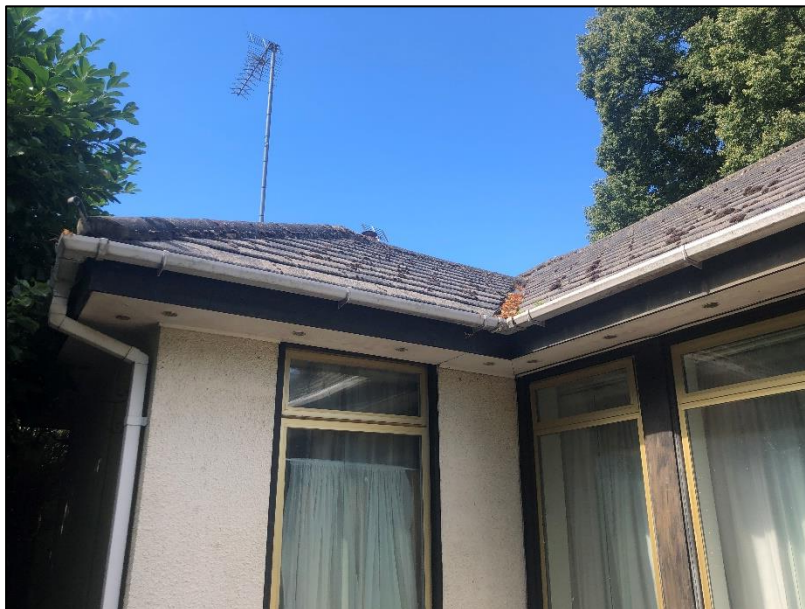
Plate 5. Showing an example of tightly fitting roof tiles and soffits
