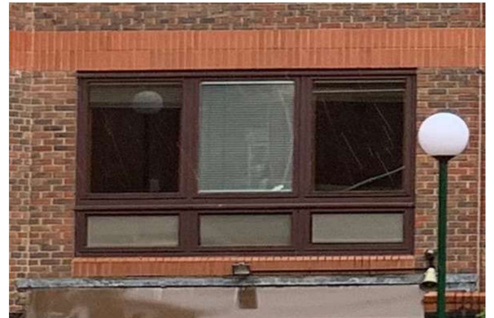
4. Existing ground floor window type
