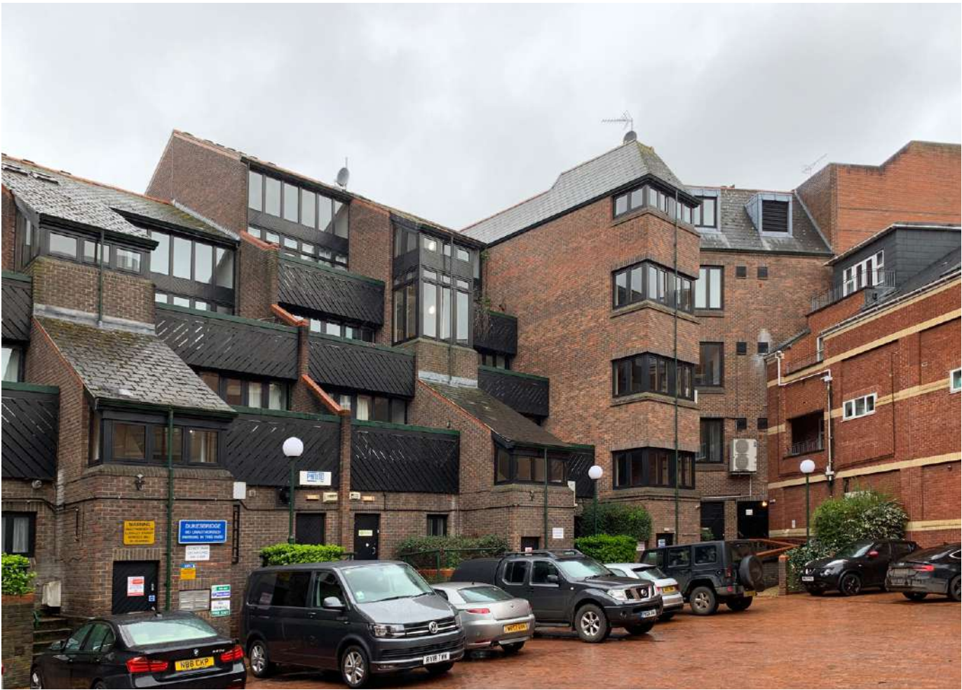
View 4 - Looking towards neighbouring buildings from the courtyard
