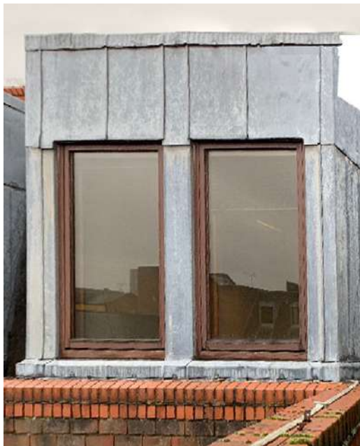
1. Existing roof level window type
