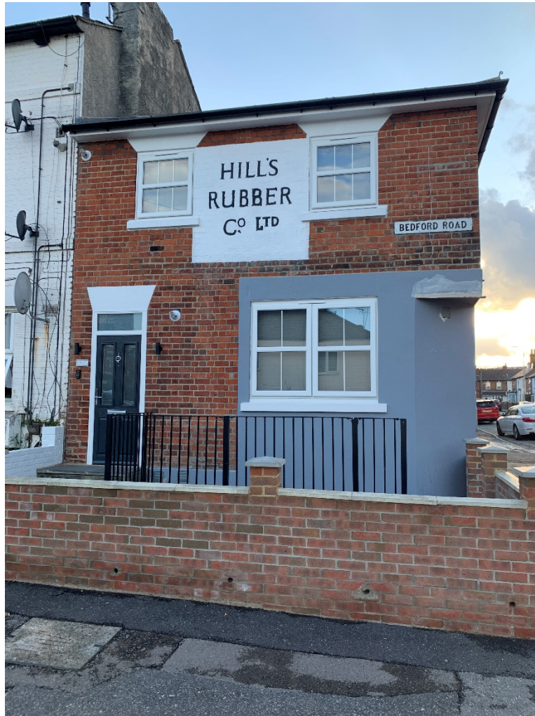
Front to Bedford Road, raised cill level to 1 st floor windows, and blanking off of corner window
