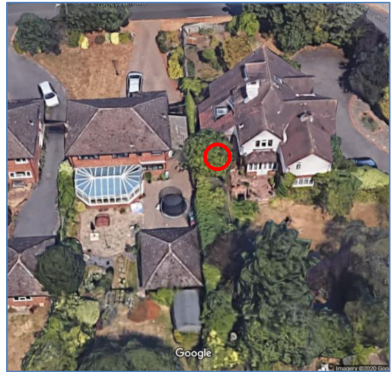
Fig 2. Aerial photo of rear of 25 Grosvenor Road in relation to 27 Grosvenor Road. Window to habitable room circled in red. (image obtained from Google Maps on 25/08/2020)
