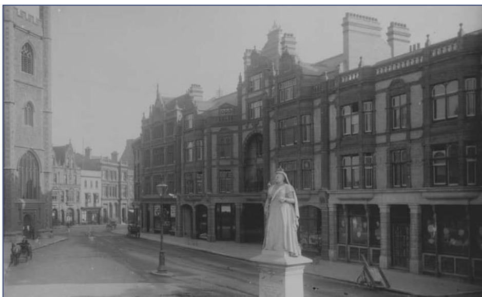
Figure 29 - Photograph dated 1893, showing the previous buildings at Nos. 173-4 and No. 175 Friar Street
