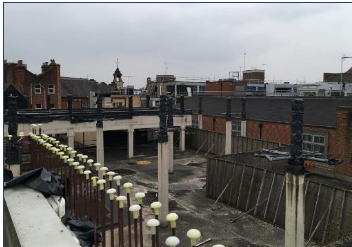
Figure 17 – Construction works to the rear of the arcade
