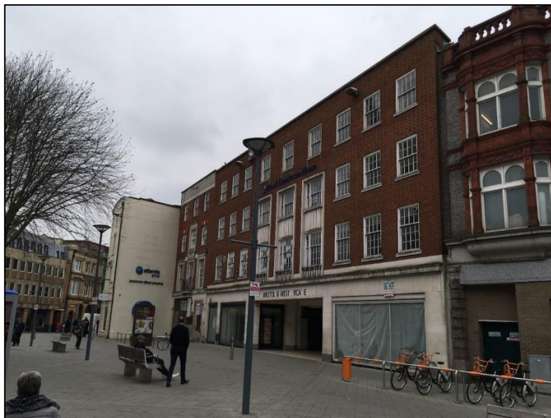
Figure 36 – Existing Friar Street elevation in March 2016
