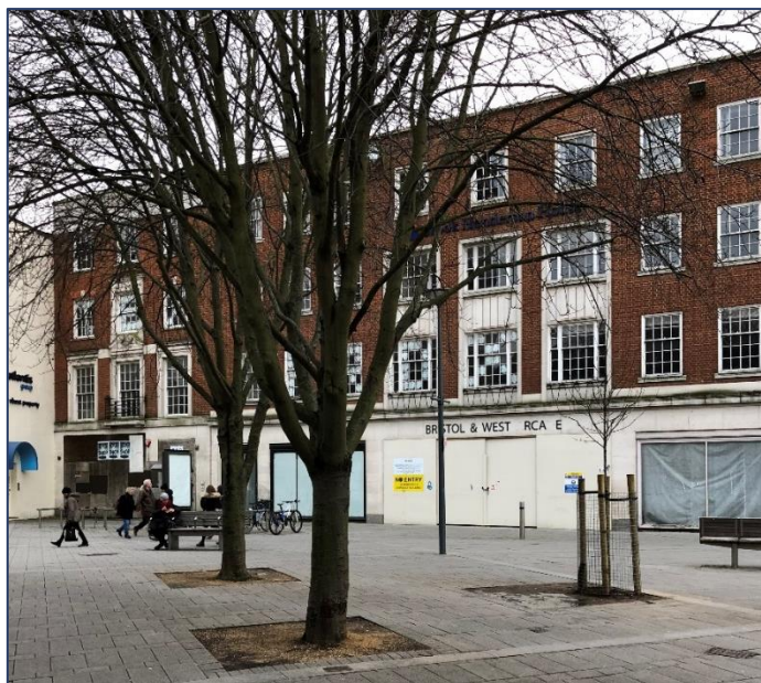
Figure 4- Existing Friar Street building
