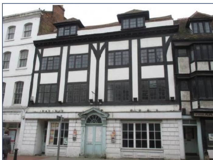
Figure 7 – 29 – 31 Market Place (Former Cooper's Arms)
