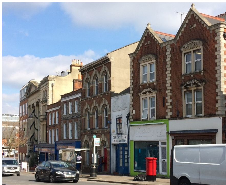
No. 43 and adjacent buildings in London Street
