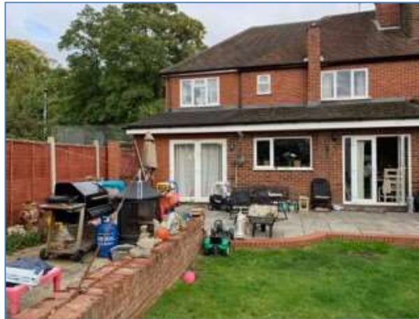
1. Existing rear elevation of 35 Honey End Lane.
