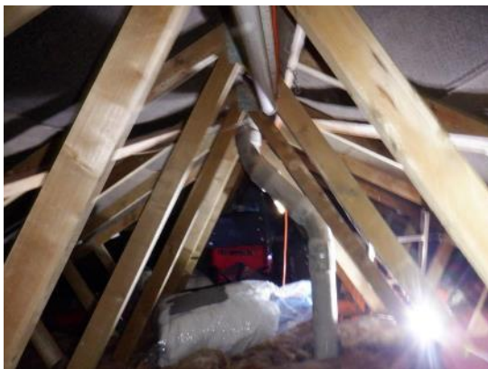
13. Roof void with trussed rafter construction.
