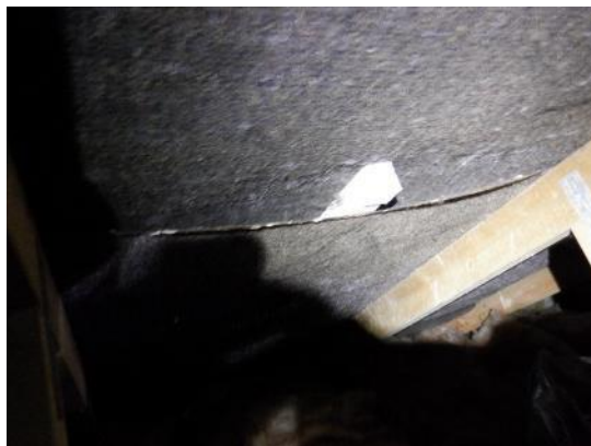
14. Hessian and bitumen felt covering roof, with pieces of polystyrene between the layers.
