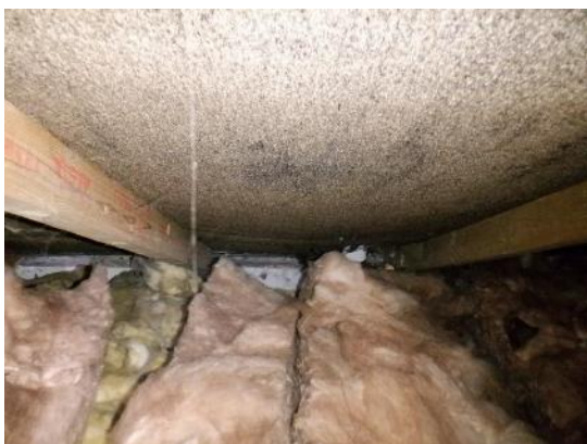
17. Open eaves and top of wall plate visible on the western side of the void.
