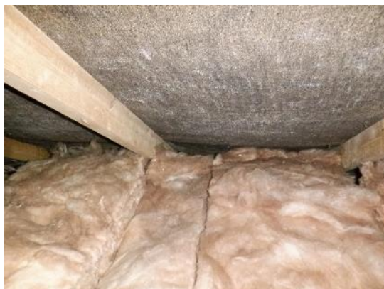
16. Eaves filled with fibreglass insulation on eastern side of the void.
