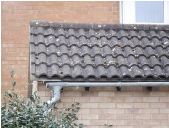
3. Tight interlocking S-shaped roof tiles.
