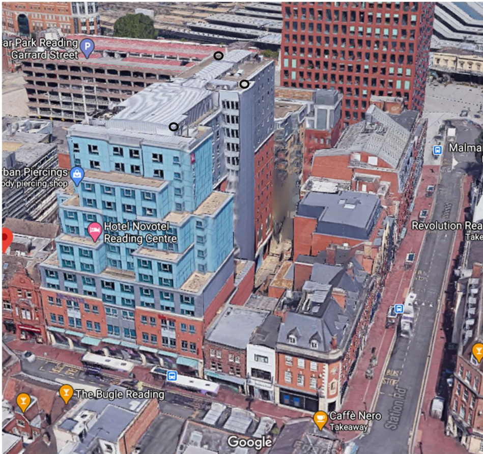
Figure 3. 3D image of application site – antenna clusters layout approximately denoted. Map source: Google.
