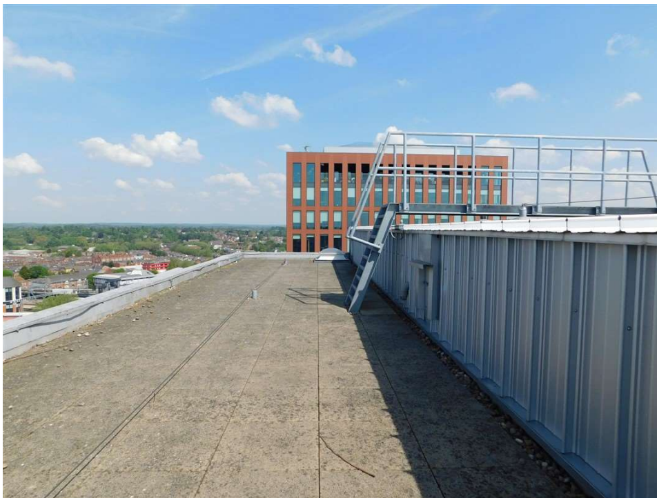
Figure 4. Photo of host building's rooftop to accommodate antennas nearest Garrard St
