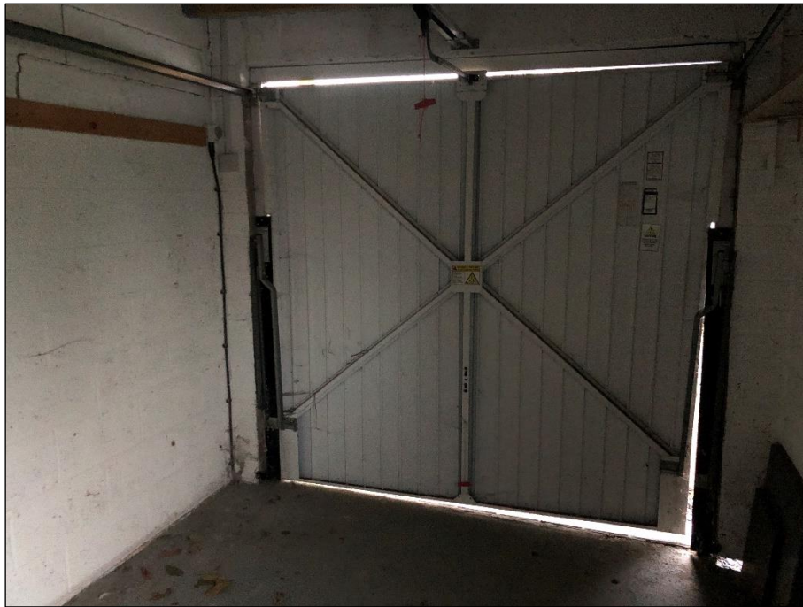
Plate 5. Interior of garage
