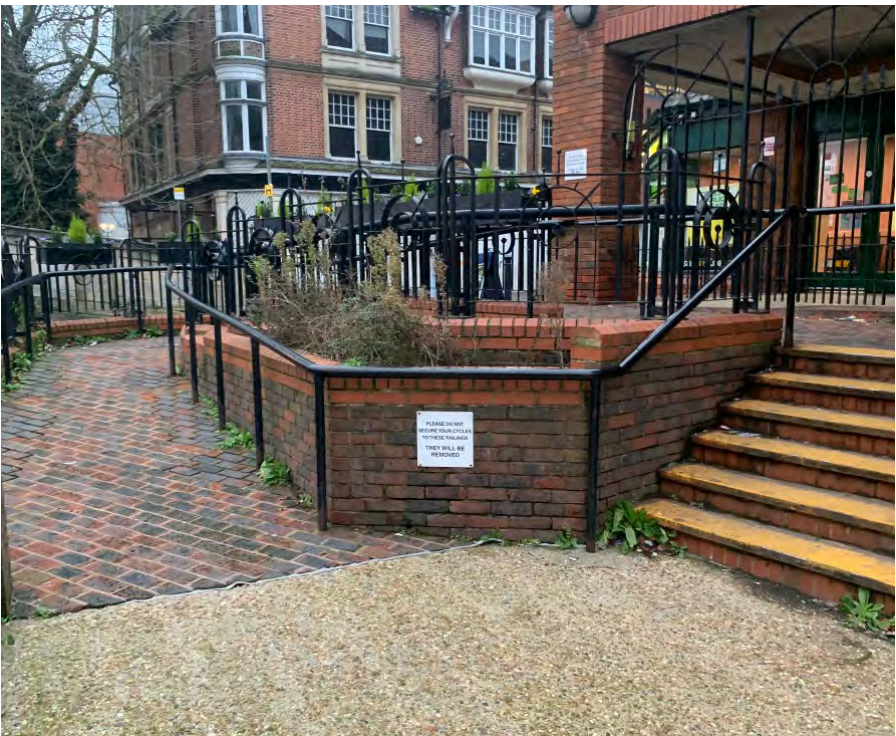
4. View of the existing ramps corner
