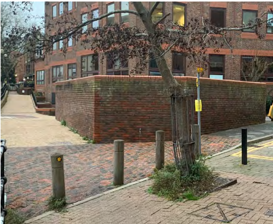
6. High substation wall providing no outlook and obstructing views from corners
