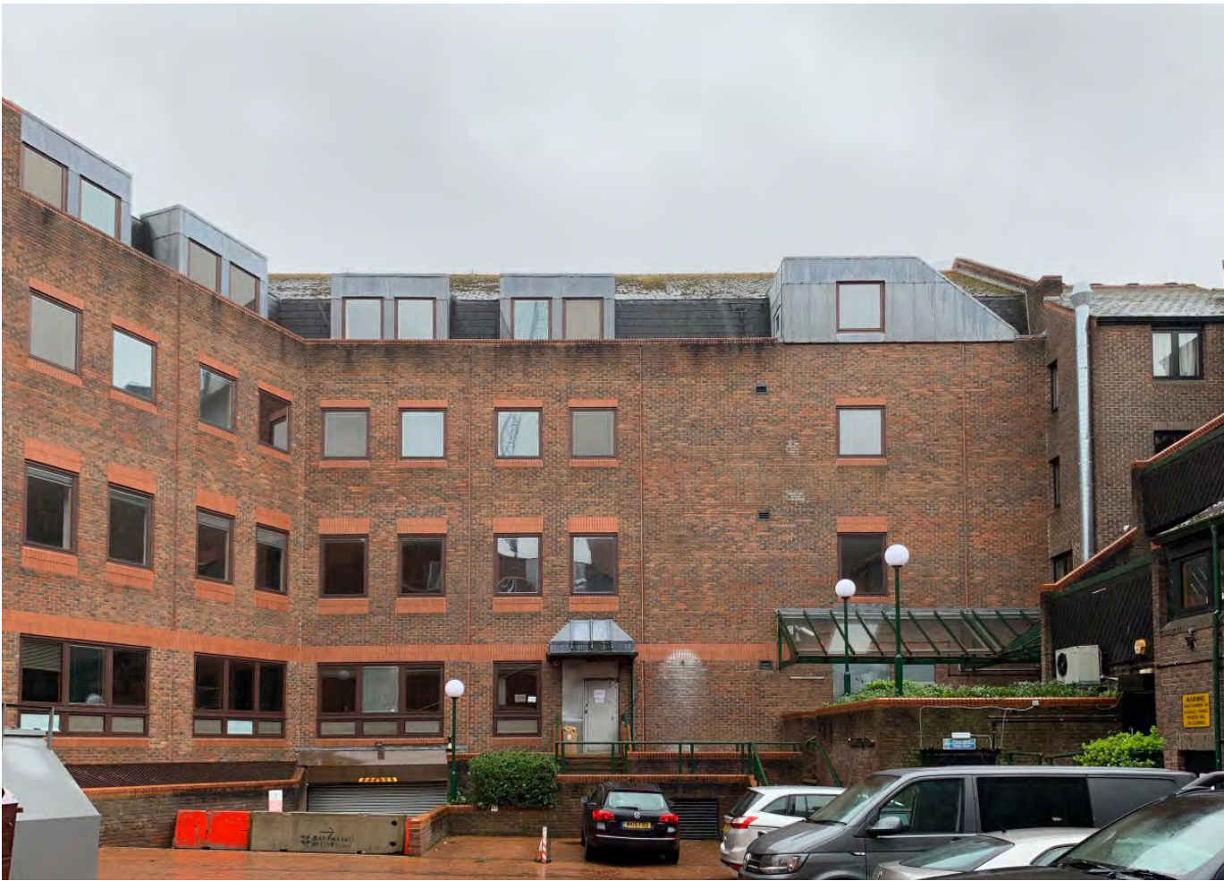
View 3 - Looking towards Dukesbridge House from the courtyard
