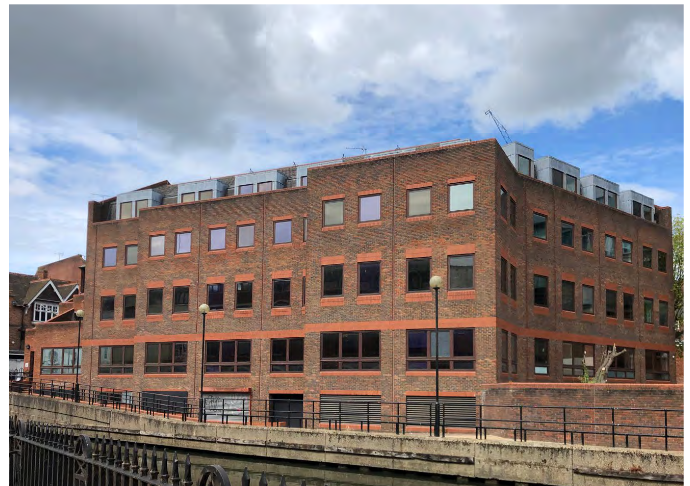
View 2 - Looking towards Dukesbridge House from the other side of the River Kennet
