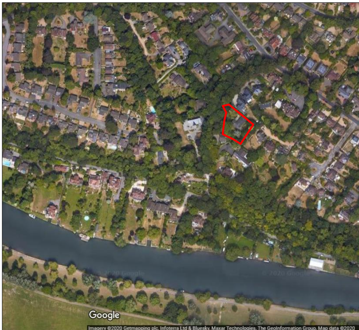
Figure 2. Overview of the site and surrounding area (the demolished building is still present within the overhead image)
