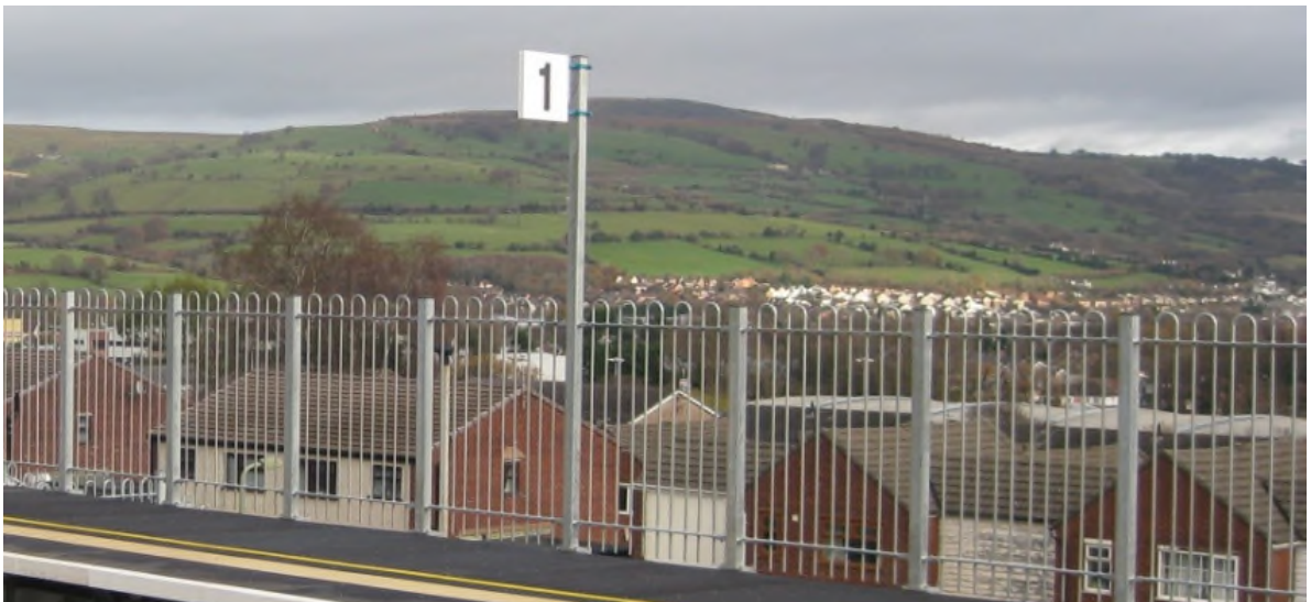
Safety top fencing
