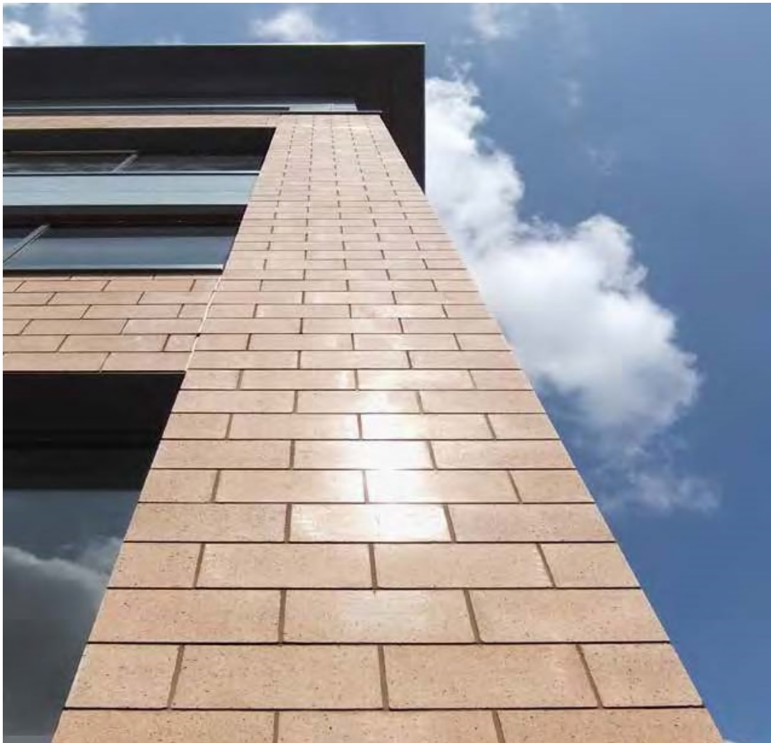
Photograph showing the 'burnished venezia' finish to the Forticrete blocks.
