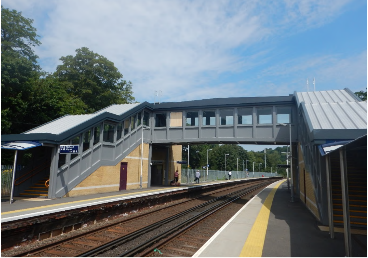
Godalming Bridge & Staircase
