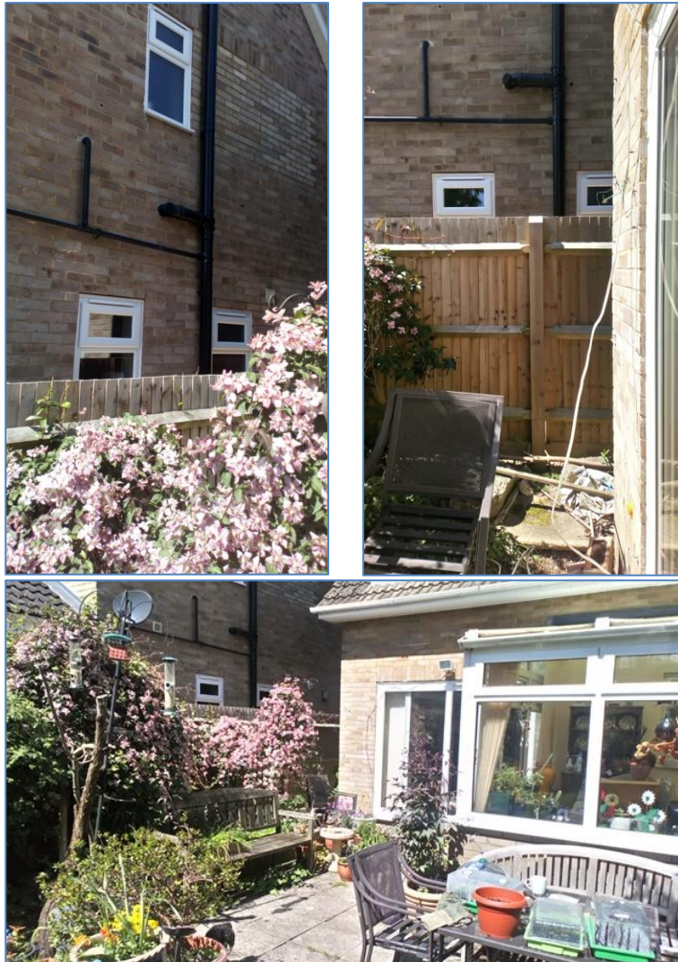
2. Windows to the side elevation of 38 Silverthorne Road. Photos received from agent on 07/05/2020
