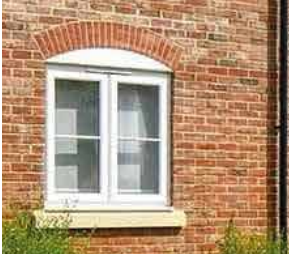
White pvc low maintenance casement style windows with horizontal glazing bar, matching white pvc rear french doors.
