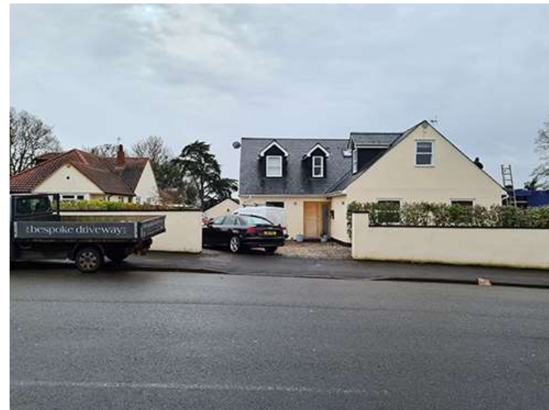
Existing frontage of dwelling
