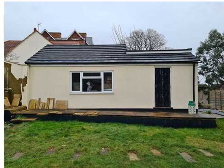
Existing side boundary (north)
