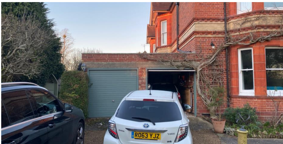
Existing Garage with doors 2m wide suits only small cars.
