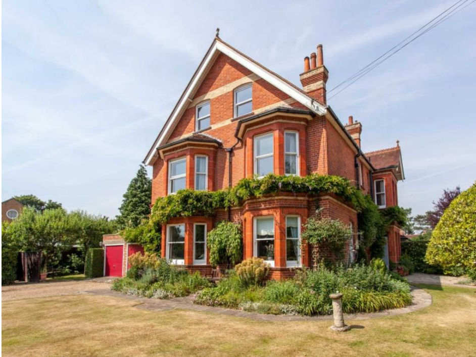
Existing South Elevation photograph with garage beyond
