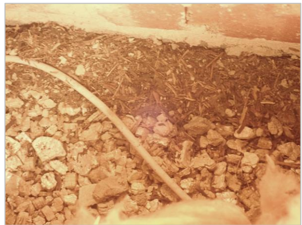
Photo 10 Spot check under modern insulation
