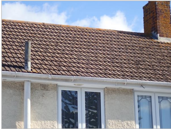
Photo 13 Roof and ridge tiles in good condition
