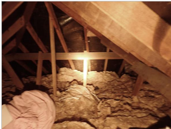
Photo 3 General conditions in loft (hipped gable end)
