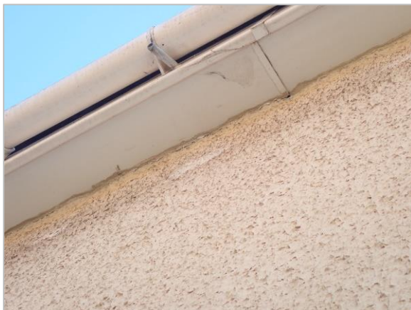
Photo 17 Soffit in good condition
