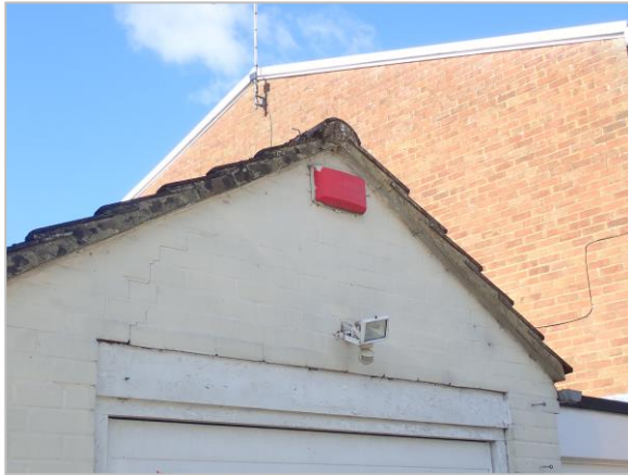
Photo 19 Garage roof in good condition
