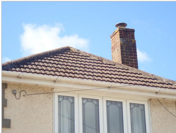
Photo 15 Roof and ridge tiles in good condition
