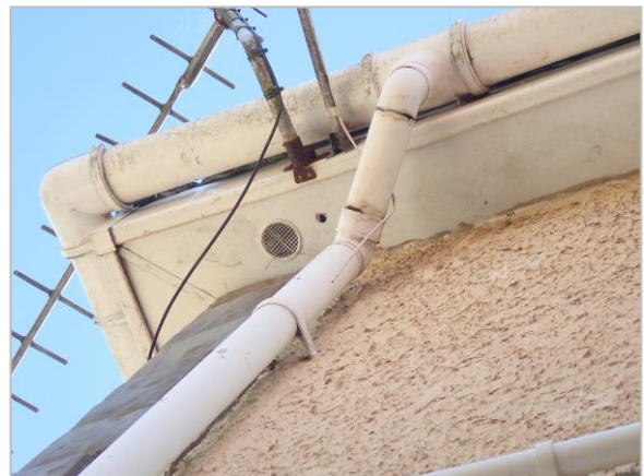
Photo 18 Soffit in good condition
