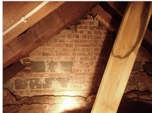
Photo 4 General conditions in loft (partition wall)
