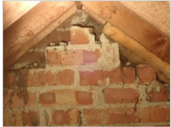
Photo 8 Brickwork partition wall
