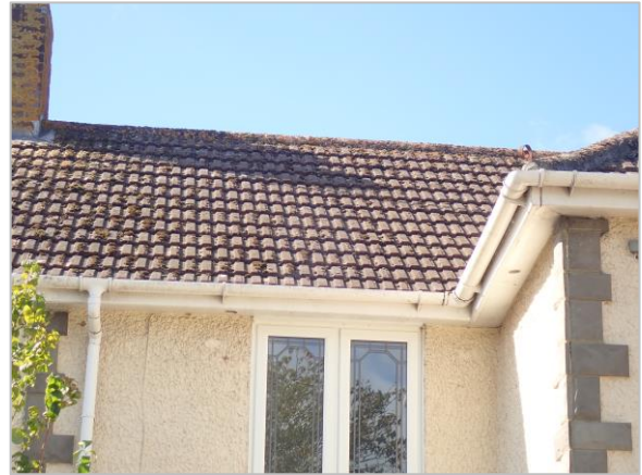
Photo 14 Roof and ridge tiles in good condition
