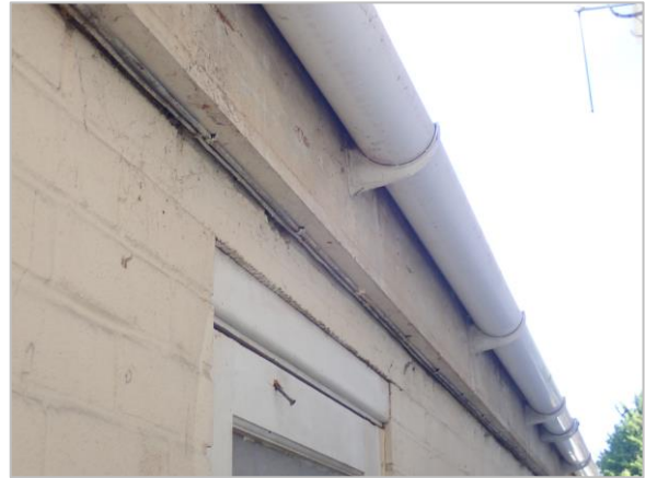
Photo 20 Fascia around garage
