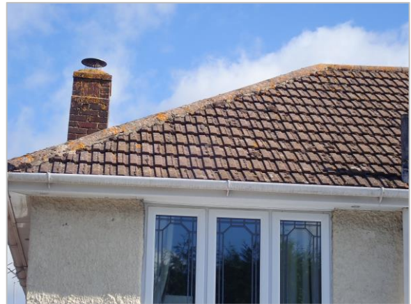
Photo 16 Roof and ridge tiles in good condition
