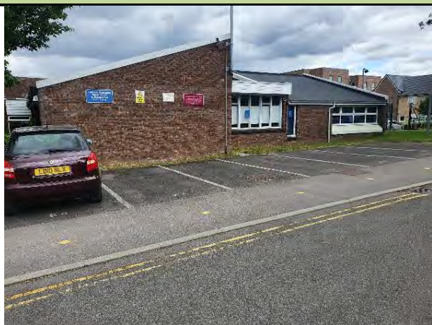
Photo 1: School buildings and car park in northern section
