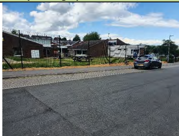
Photo 2: School buildings and soft landscaping in northern section
