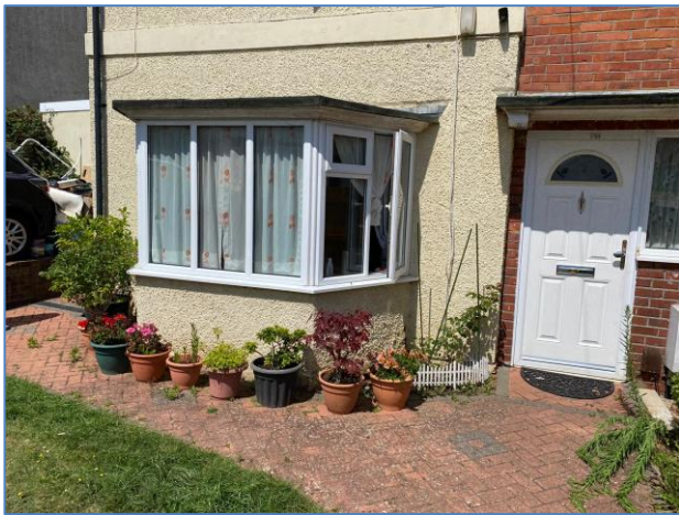
1. Front of 2 Ripley Road. Photo provided by the agent on 15/08/2020.
