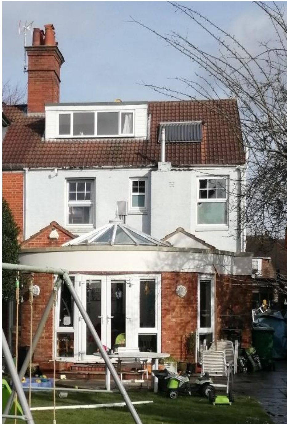
Fig 4. Photo of rear elevation
