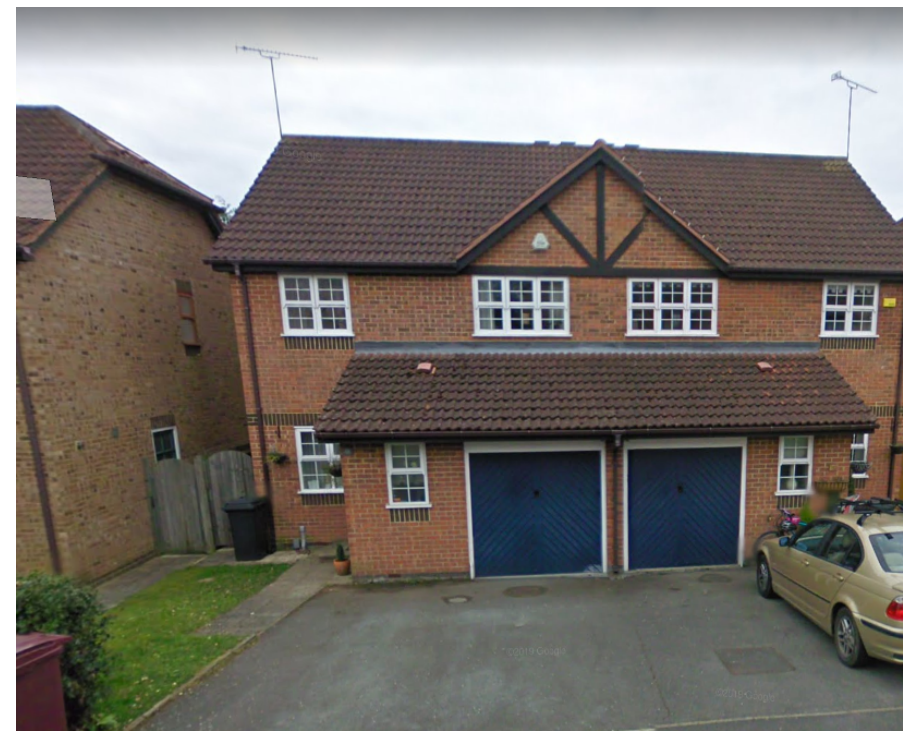
Existing Front Elevation Photo
