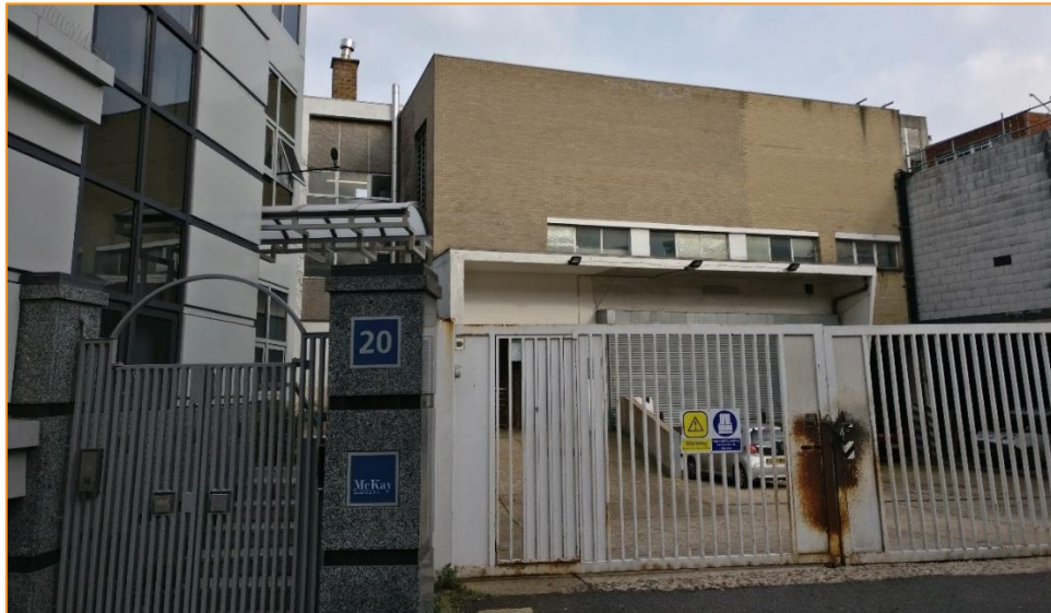
Figure B.3: Photographs of MP3
