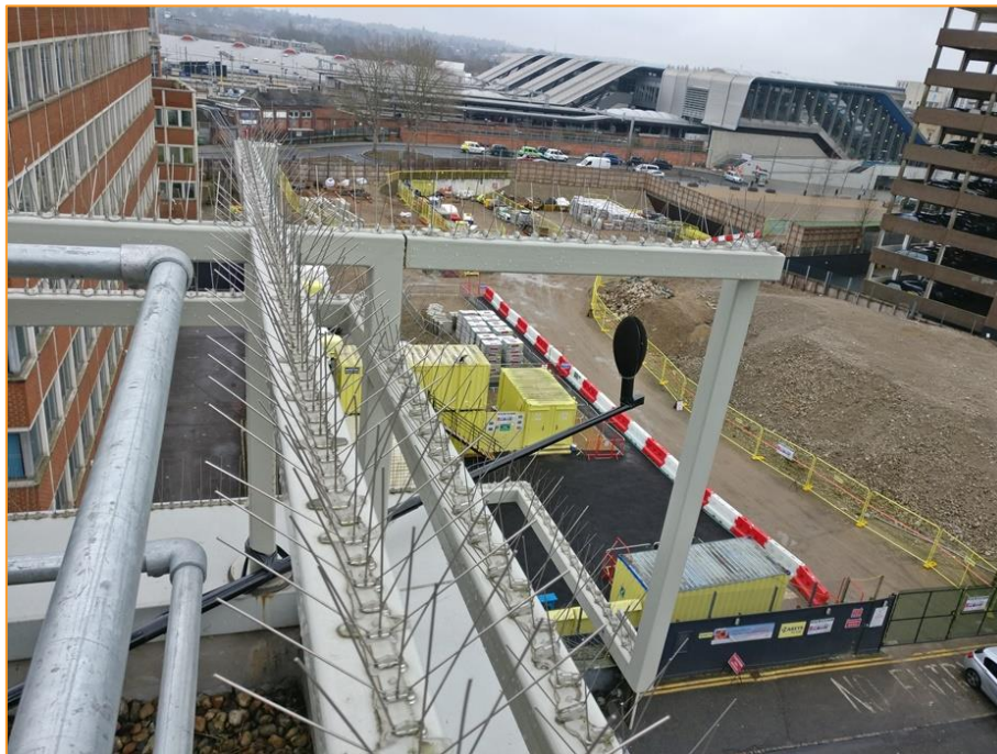
Figure B.2: Photographs of MP2
