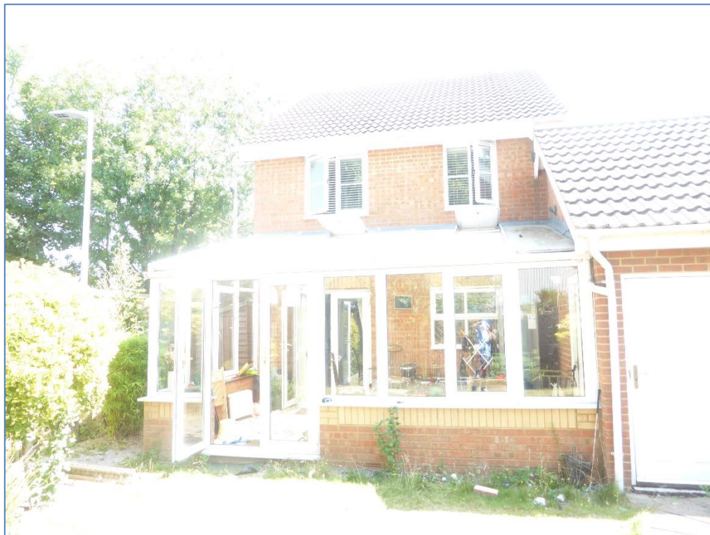
1. Existing conservatory at 31 Denbeigh Place (image supplied by agent).
