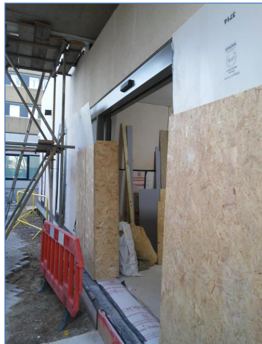
2. Partially constructed entrance to proposed extended entrance lobby. Photo supplied by agent on 13/01/2021
