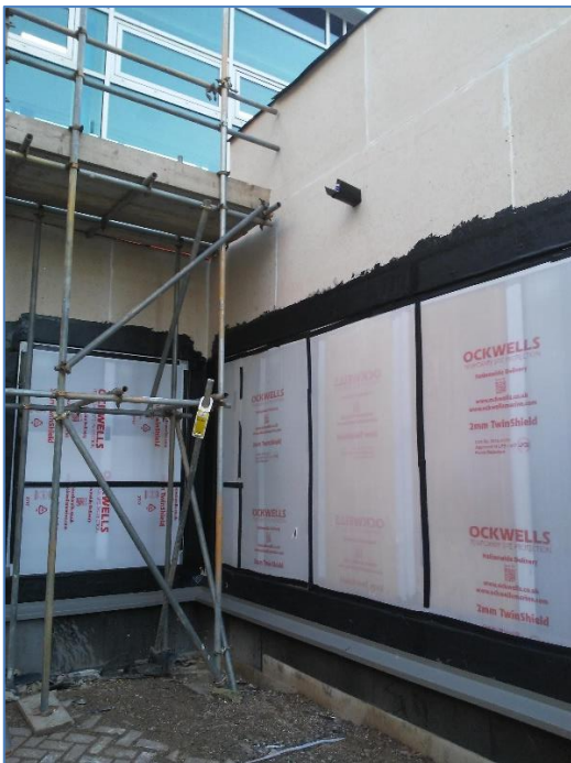
1. Side elevation to partially constructed entrance lobby, looking south. Photo supplied by agent on 13/01/2021
