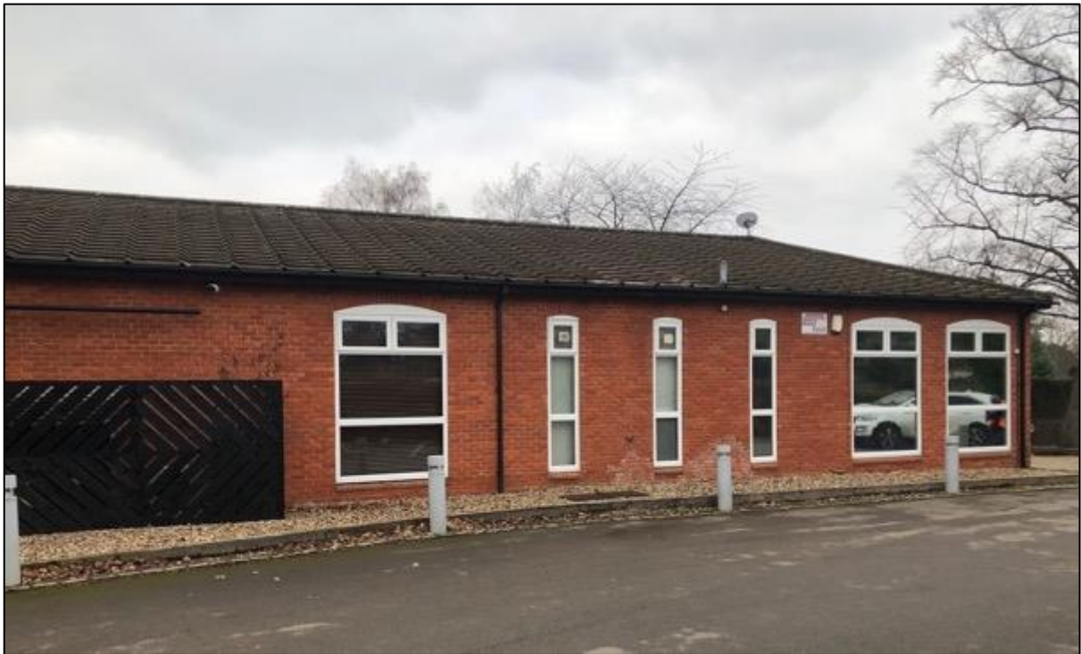
Photograph 1. The clubhouse at Reading Golf Club viewed from the east.
