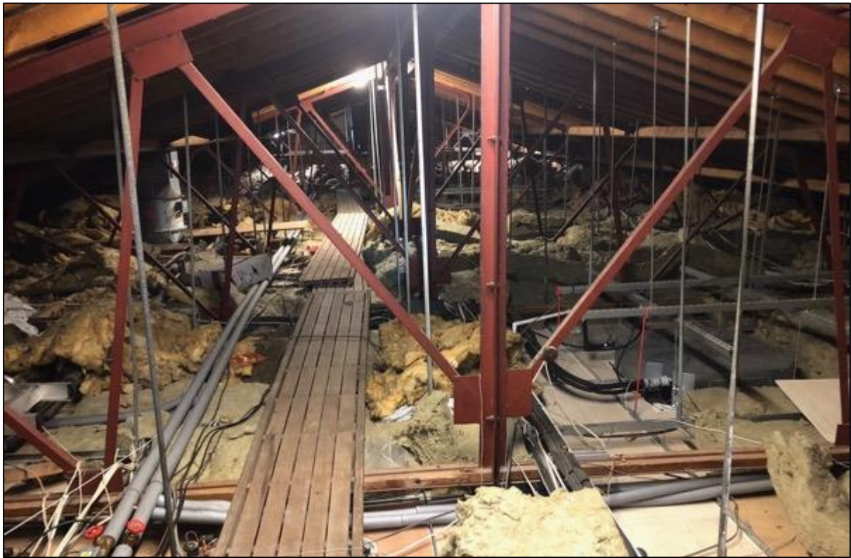
Photograph 3. The loft space within the clubhouse.
