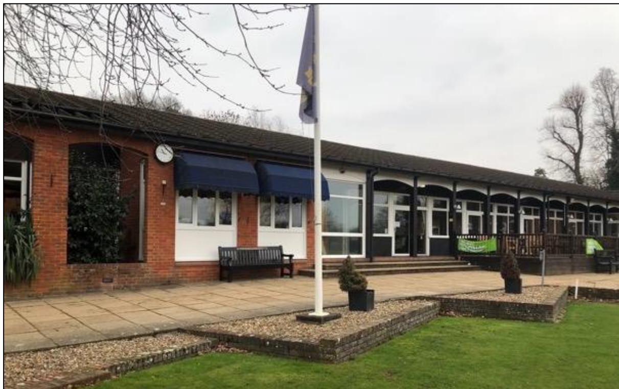
Photograph 2. The western elevation of the clubhouse.
