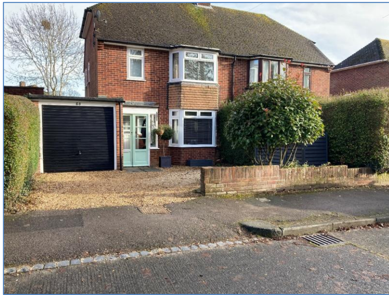
1. Front of 68 Surley Row. Photo provided by applicant on 23/01/2021.
