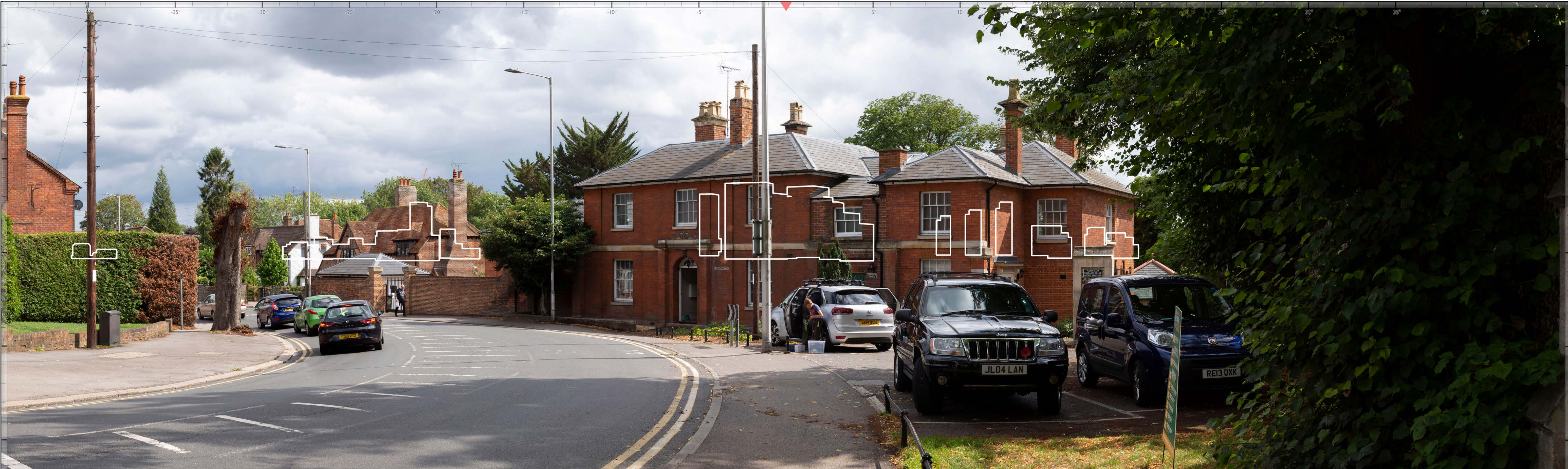
View 22 Church Road by Caversham Court looking SE - Existing
