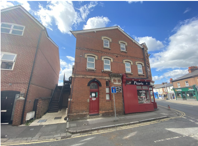
Figure 7: View of side elevation of 5 Prospect Street
