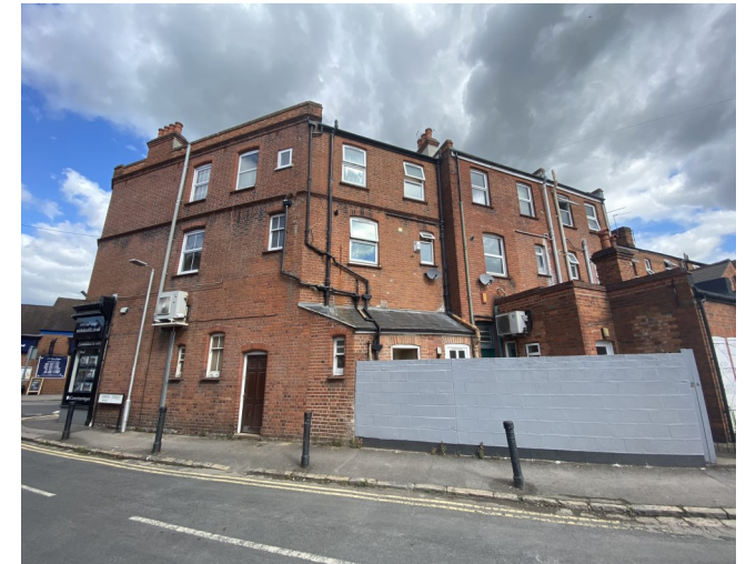
Figure 9: View of side and rear elevations of 7 Prospect Street
