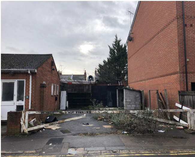
Figure 4: Dropped Kerb to be reinstated and gate removed
