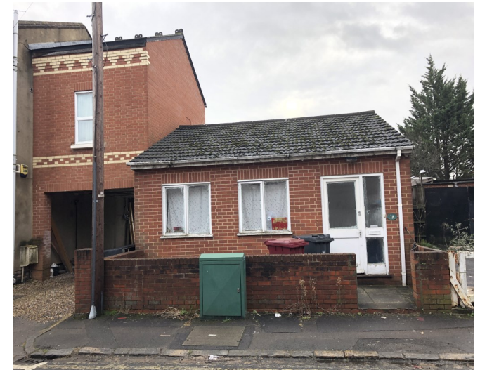
Figure 6: Bungalow to be demolished
