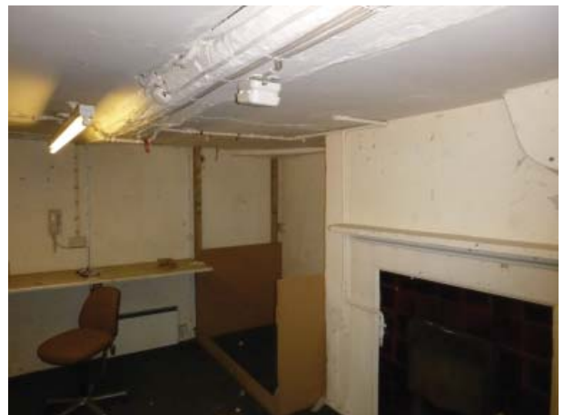
Plate 6. Basement of 27-28 Market Place - 'Kik Sports'
