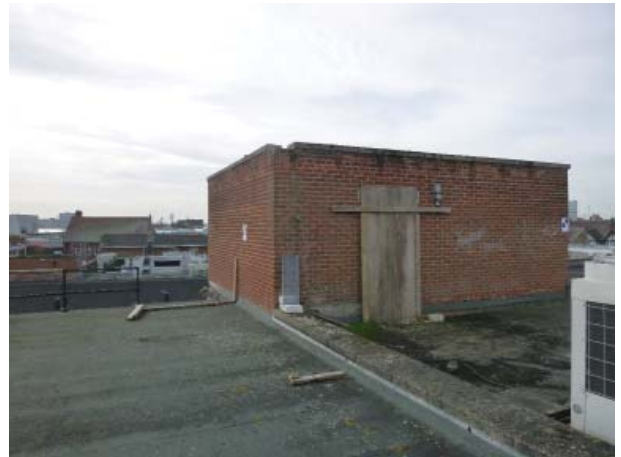
Plate 4. Roof and small external structure/room of 173-175 Friar Street - 'Bristol and West Arcade'
