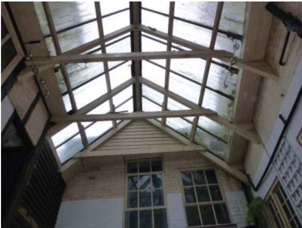
Plate 15. Pitched glass roof above former pub within 29-31 Market Place 'Coopers Arms'
