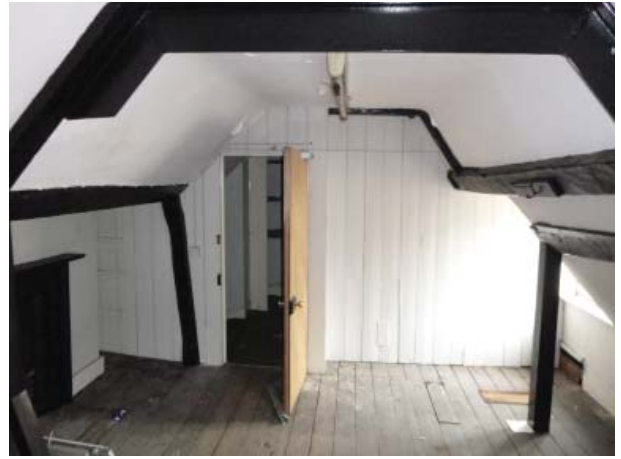
Plate 8. Third floor of 27-28 Market Place - 'Kik Sports' with dormer windows
