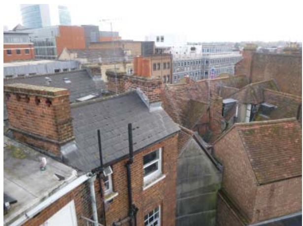
Plate 24. Roof structure of 27-32 Market Place
