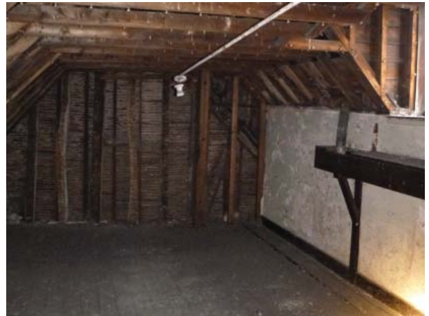
Plate 16. Roof void of 29-31 Market Place 'Coopers Arms'
