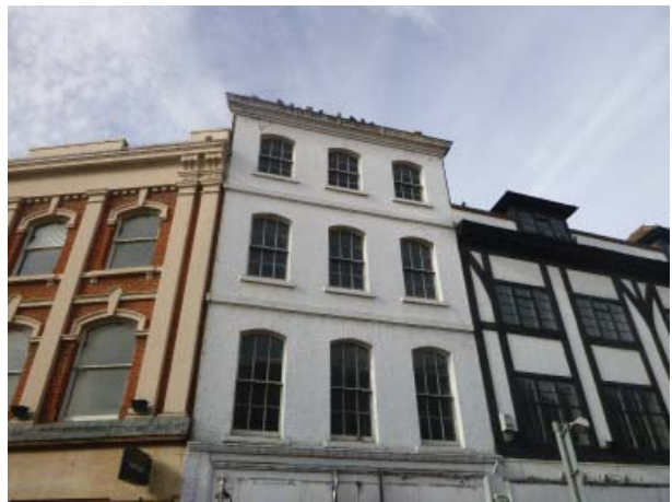
Plate 20. Exterior of 32 Market Place (upper levels, not accessed during survey)
