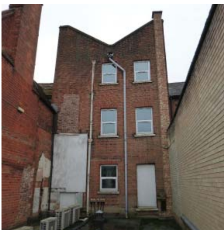
Plate 23. Rear exterior of 32 Market Place (interior of these levels not accessed during survey)
