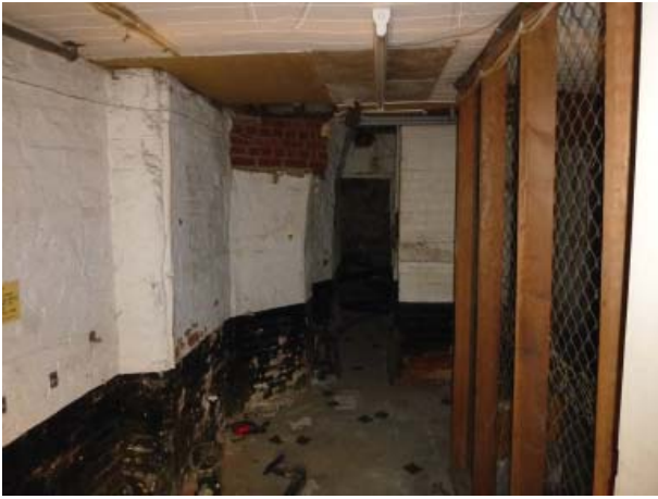
Plate 13. Basement of of 29-31 Market Place 'Coopers Arms'
