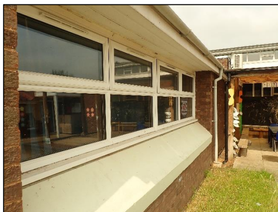
Photo 20 Soffit box. Building to north east of site.
