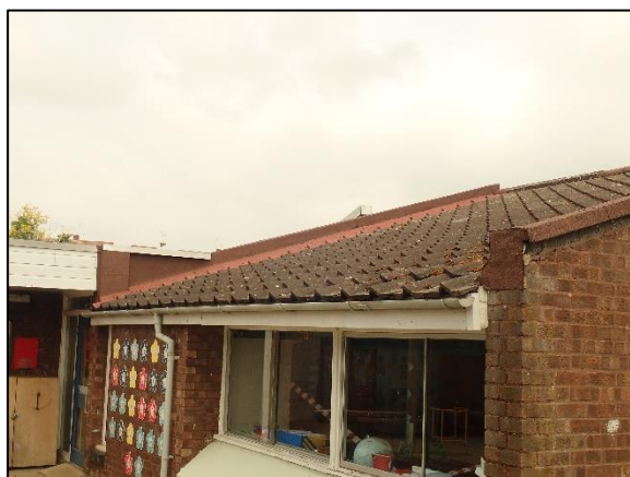
Photo 19 Interlocking concrete pantiles. Building to north east of site
