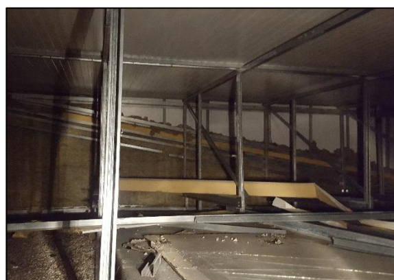
Photo 16 Interior void of over-roofed section
