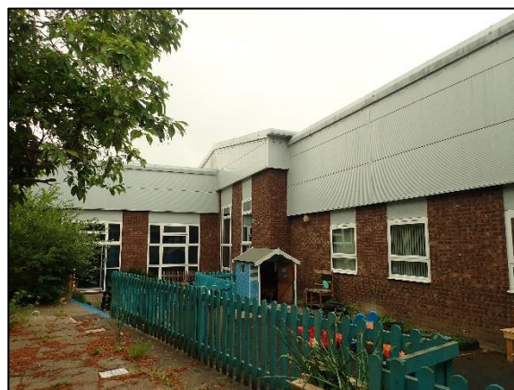
Photo 14 Over-roofed section of building – exterior view
