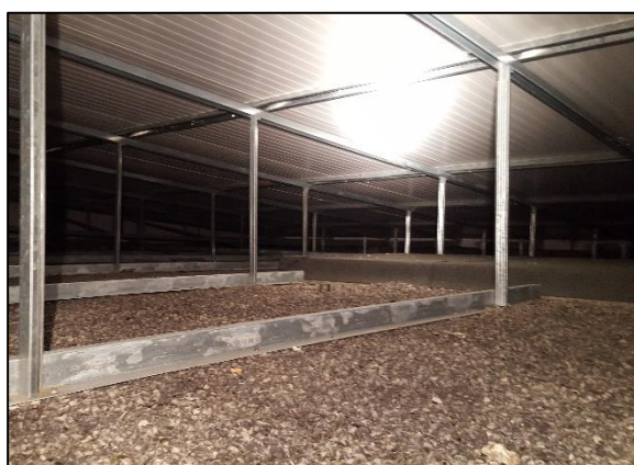
Photo 15 Interior void of over-roofed section
