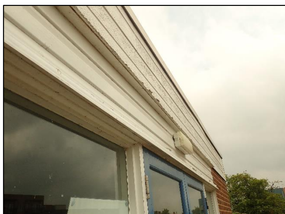
Photo 17 Timber weather boarding on building to north-east of site
