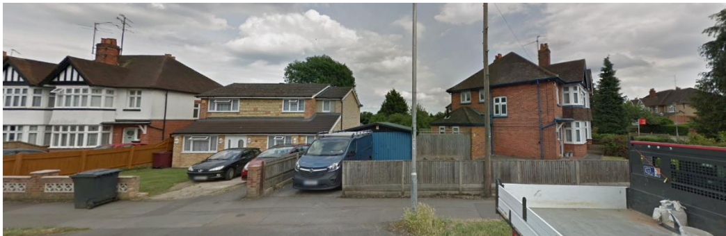
Image: Google Maps. No. 15 is located on the right, at an angle to the road, no. 15A to the left with the existing garage in between
