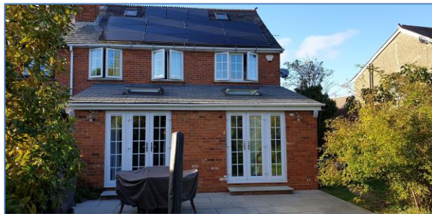
Fig 3. Site photo (rear elevation) provided by applicant on 08/09/2020.
