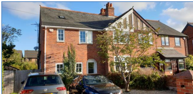
Fig 1. Site photo (front elevation) provided by applicant on 08/09/2020.
