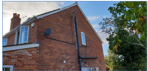
Fig 2. Site photo (side elevation) provided by applicant on 08/09/2020.
