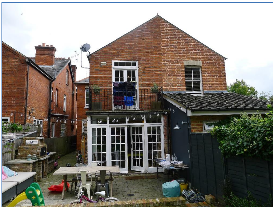
1. Rear of 3 St. Anne's Road. Photo provided by the agent on 13/11/2020.
