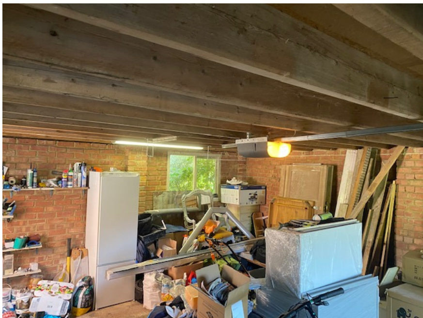
Photo. 3 Internal exposed roof joists
