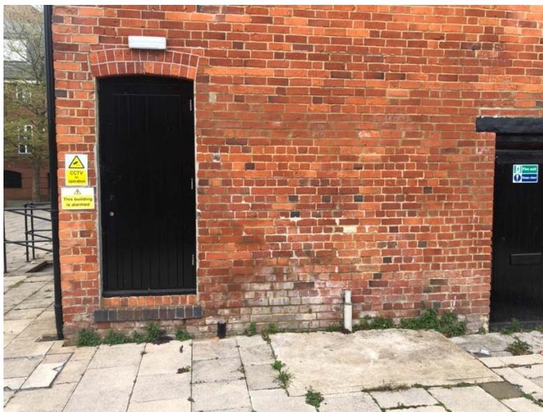
Fig 1 – Comparison West elevation, before and after restoration works.
