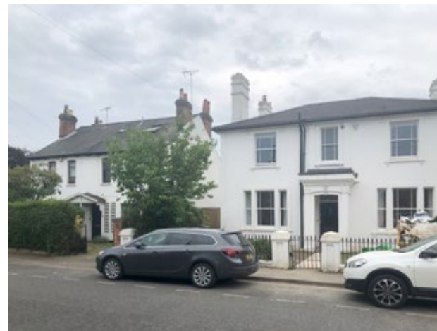
VIEW TO 43/39 UPPER REDLANDS ROAD SHOWING BLACK WINDOW FRAMES TO NO. 39
