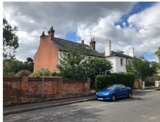
VIEW TO 43/39 UPPER REDLANDS ROAD SHOWING BRICK FLANK WALL TO NO.39
