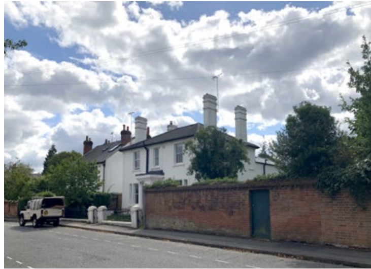
EXISTING STREET VIEW
