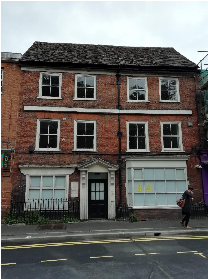
Fig 1: As viewed from Gun Street (2019)
