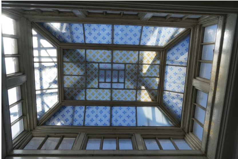
Skylight with applied colour glazing (01565)
