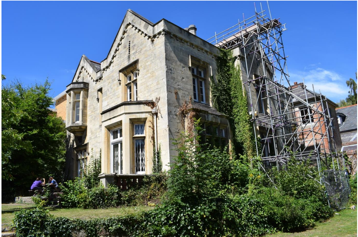
View of the south and east elevations (049)
