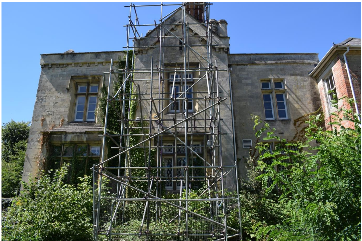
View of the east elevation showing the change in detail to the RHS of the gable and the brick wing (052)
