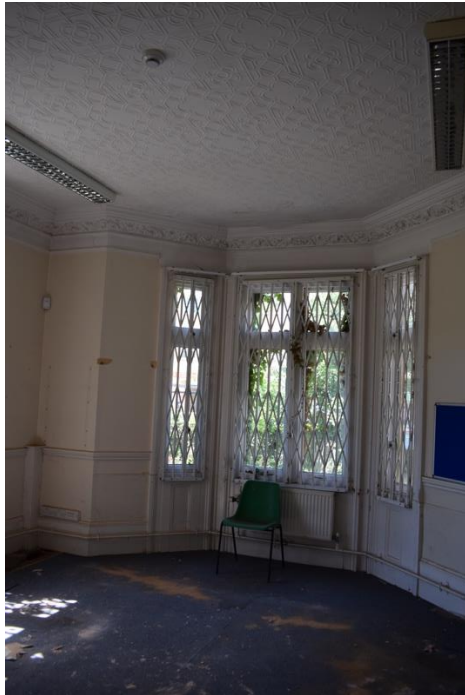
Decorate plaster ceiling and cornice (0030)
